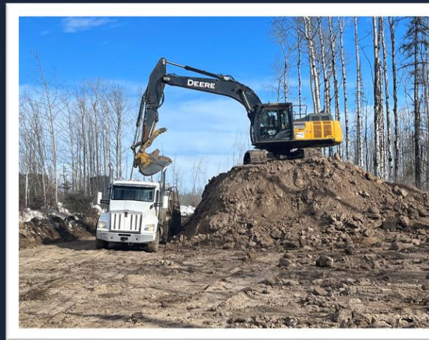
LOADING CLEAN BACKFILL
